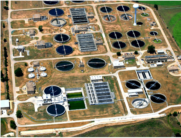
South Austin Regional Wastewater Treatment Plant
